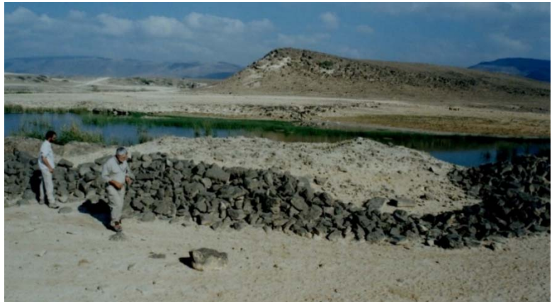
Fig. 2 - The area before the works in 2006 (photo A.V. Sedov, ©IMTO)
