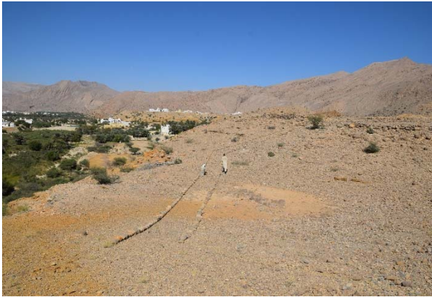
Fig. 5 - The building of the visitor pathways, from the wall's perimeter leading toward the inner part of the site (©University of Naples L'Orientale)
