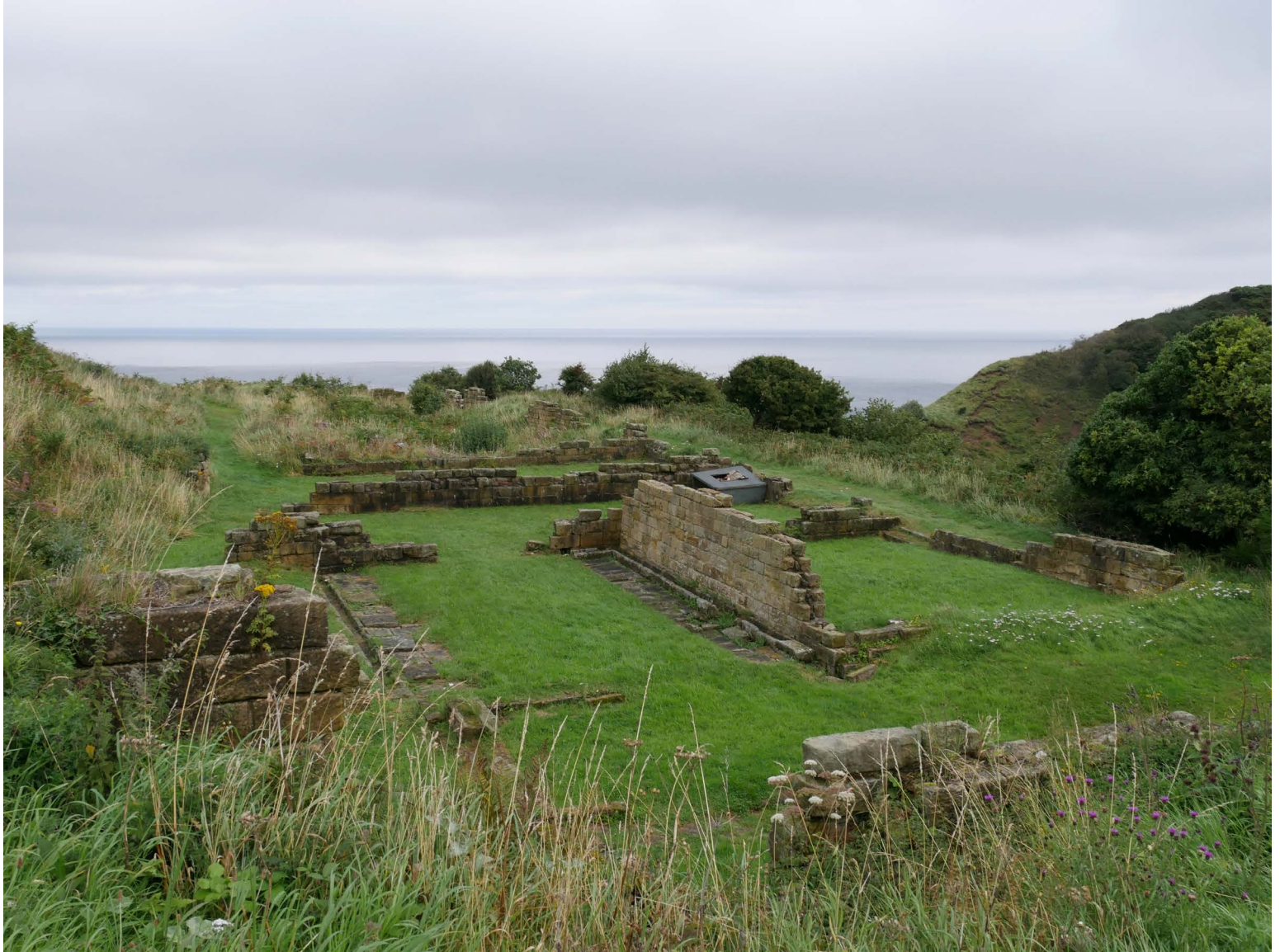
Fig. 2: Peak Alum Works, Ravenscar, North Yorkshire. 1349509 NTPL Commissioned (NTPL) ©National Trust Images/Zoe Frank.
