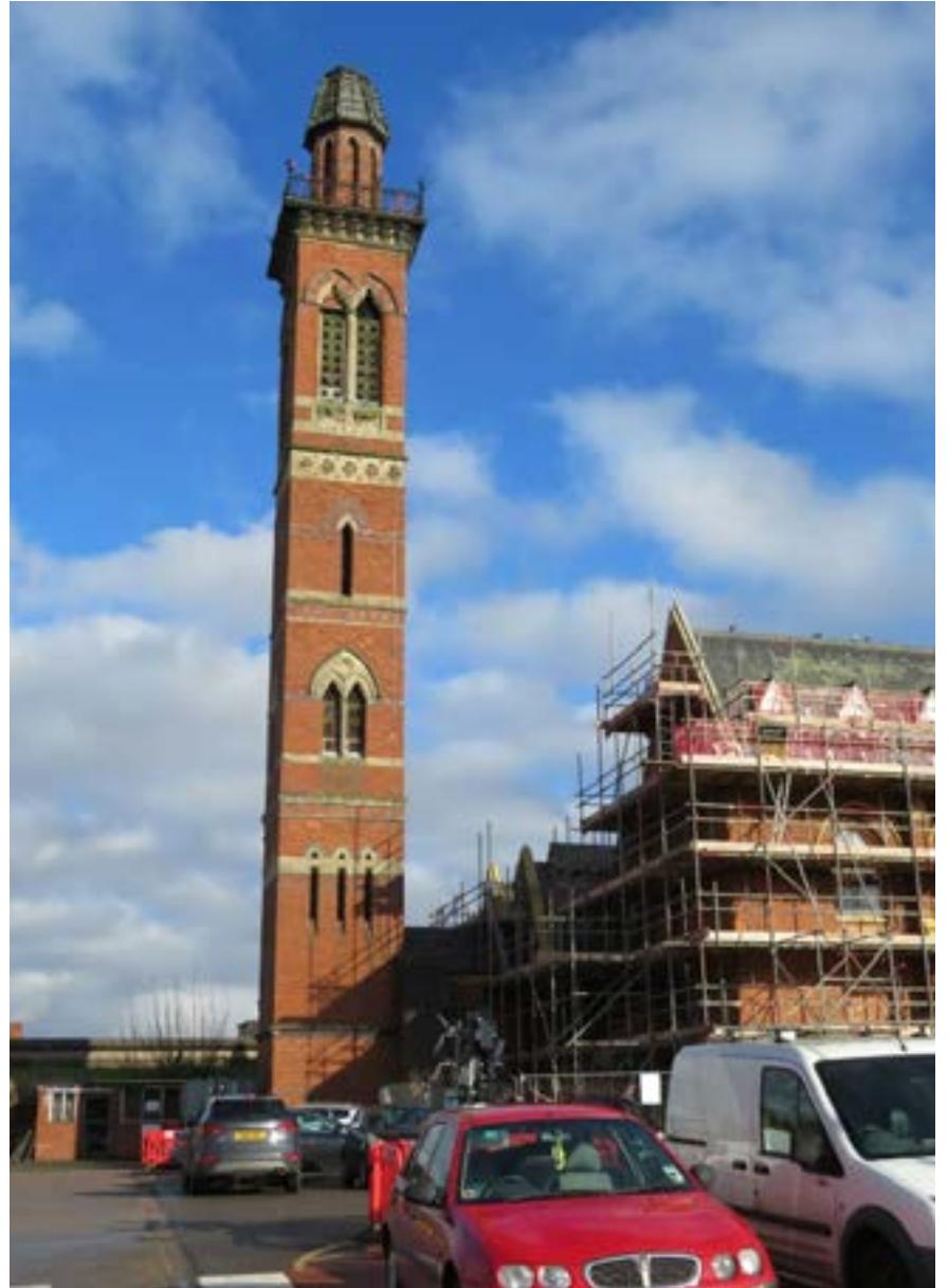
Fig. 5: John Henry Chamberlain and William Martin, Edgbaston Pumping Station, Birmingham, constructed around 1870, today.
