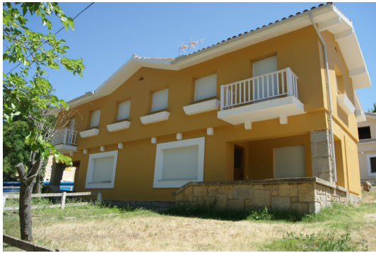
Fig. 6: Housing building in Salto del Esla in 2020 (photo by the author).
