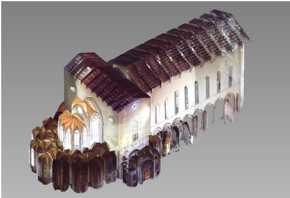
Fig. 5 - S. Lorenzo. Point Cloud from 3D laser Scanner survey
