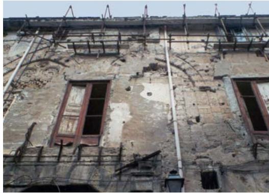
Fig. 3-4: Palermo, Cefalà Palace. The front damaged by the collapse of the façade of Palazzo Bonagia, before the removal of the plaster and recent reinstating of the surfaces (photo 3 by Giovanni Trovato, early 1990's; photo 4 by the author).
