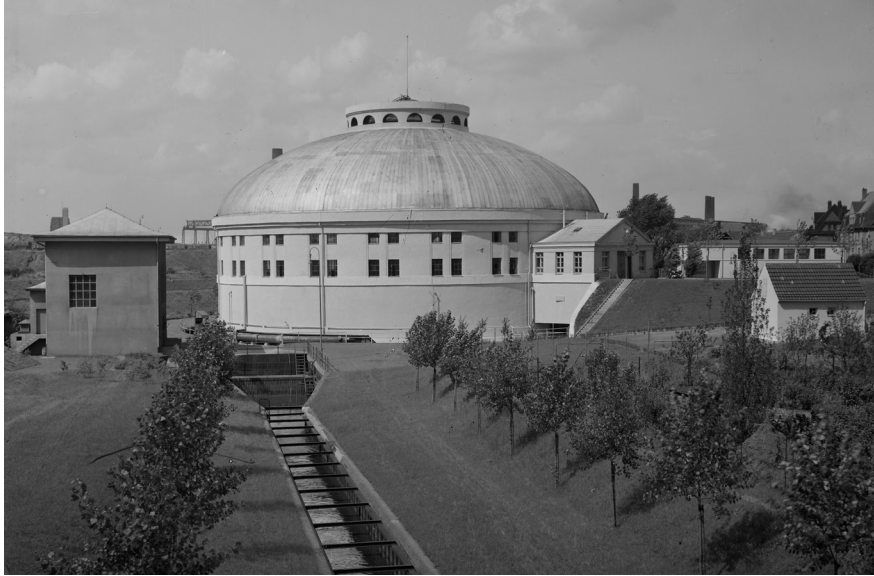
29. The Old Emscher Pumping Station in a contemporary picture, is still in operation today (Photo: Emschergenossenschaft).
