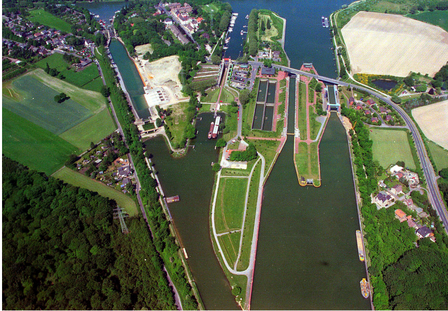
27. Over the course of 90 years, four parallel descending structures were built in Henrichenburg, including the old Ship-Lift on the left. Three of the structures are no longer in operation and are listed buildings (Photo: WSV) Photo: LWL-Industriemuseum).
