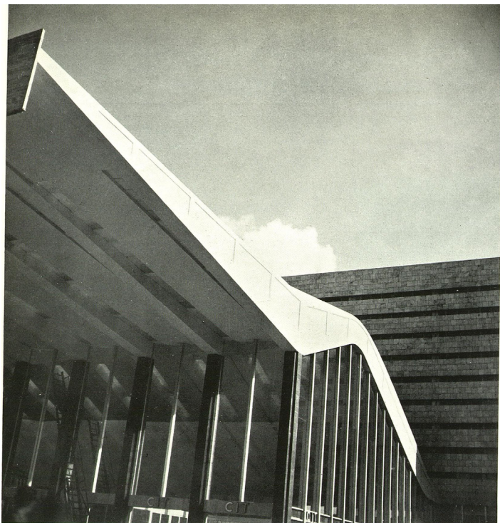
6, a detail of the reinforced-concrete roof of the booking hall which extends to form a canopy over the roadway in front of the station. Behind can be seen part of the office block. 7, general view of the booking hall and canopy. The curved shape of the beams follows the profile of the ruins of the Agger Serviano, as can be seen in 9, on the facing page.
