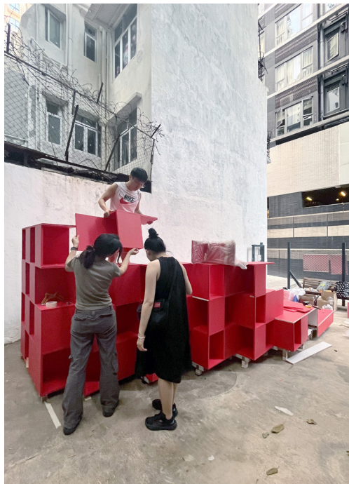
Fig. 4 - The research team assembling the project structure, built with a timber framework of 48mm section (Photo by Giovanna Santoro)
